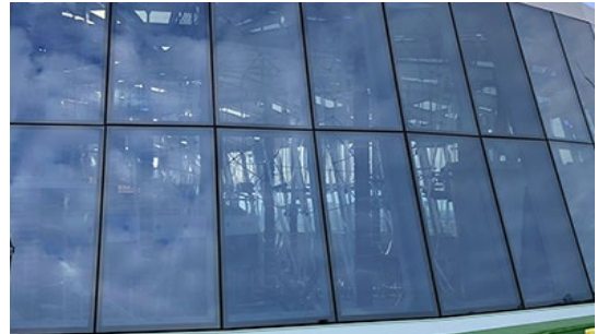
Glued fire resistant glazing No screwed frames – more flexibility in design!
