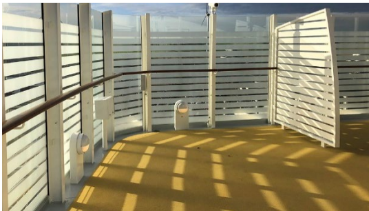
Windscreen and Railing solution Delivery of glass and steel structure!
